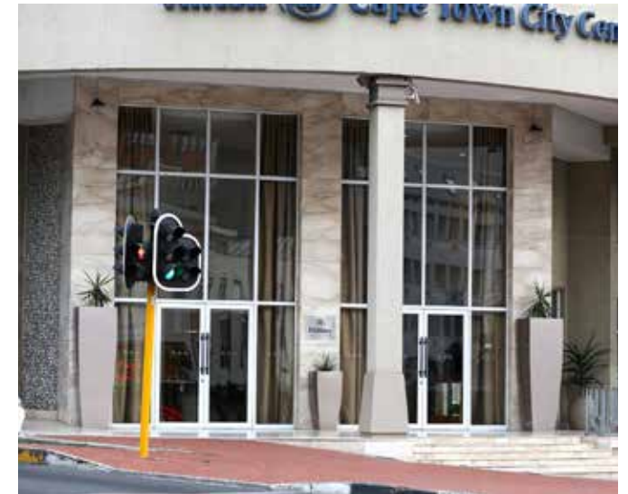
Hilton Hotel - Cape Town (project by Servest) (shown above)
